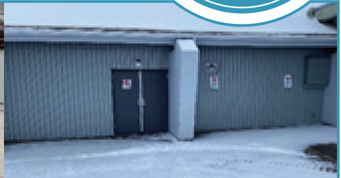
Metal Cladding Installed at i-plex
