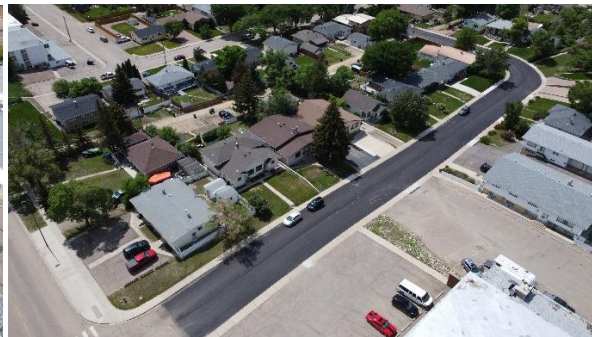
Fig. 2 Ashley Drive AFTER paving.
