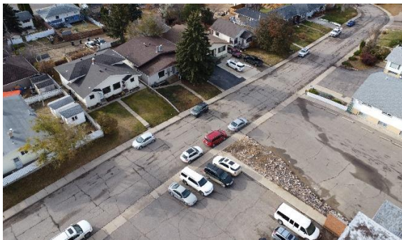
Fig. 1 Ashley Drive BEFORE paving.
