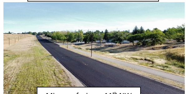
Microsurfacing – 11 th NW
