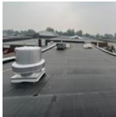
Make-Up Air Units, Aquatic Ctr
