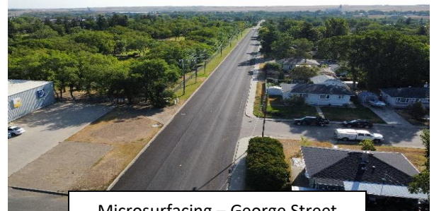
Microsurfacing – George Street
