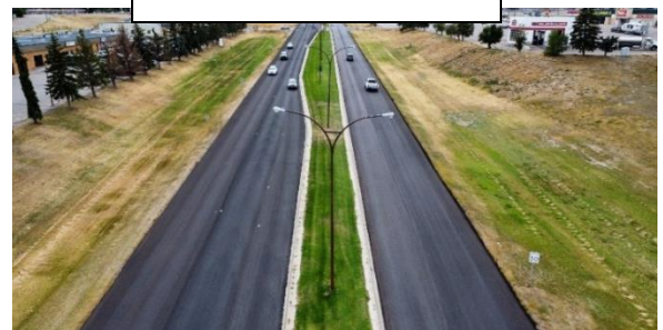
Microsurfacing (left) & Thin Asphalt Overlay (right) Central Ave N
