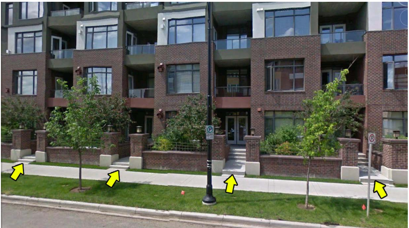
Figure 13: Ground floor apartment units with individual entrances to the street
